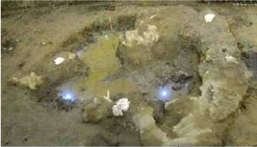
A solidified cement mass mixed with DPAA
