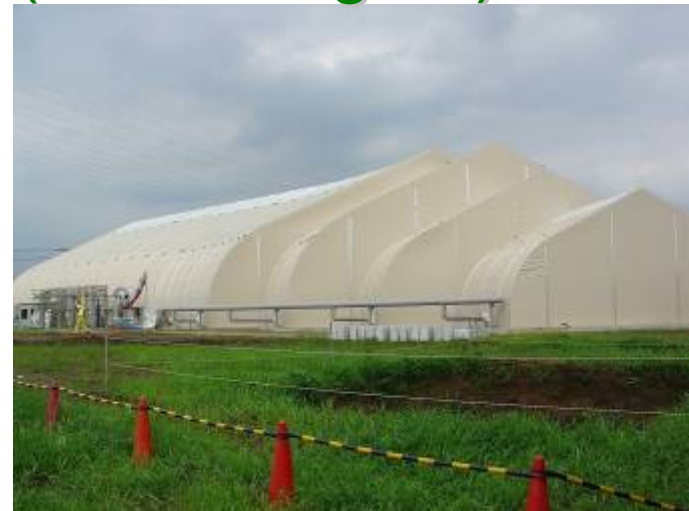
Dug-out soils were covered to prevent spreading.
